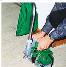
Grooving PVC and Linoleum
