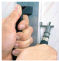
Grooving PVC and Linoleum
