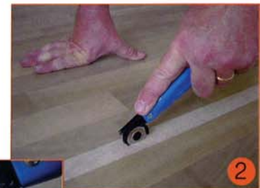
Cut masking tape easily with the rolling knife in the area of the seam. With hard coverings (e.g. object floorings) the seam area has to be heated to a maximum of 40 °C directly before welding, by using an iron or a heat gun.
