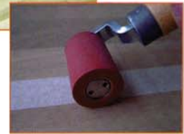
Place special masking tape centered over the closely-cut seam and press on tightly with a roll.
